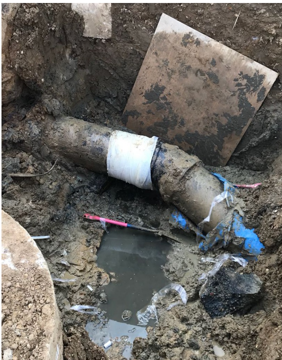
Wrap & Seal sealed the leak before overwrapping with SylWrap HD Bandage for a permanent repair
