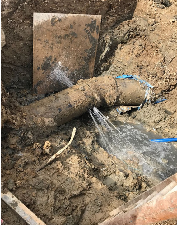
Significant amounts of contaminated water were left spraying out of the pipe after it was cut into
